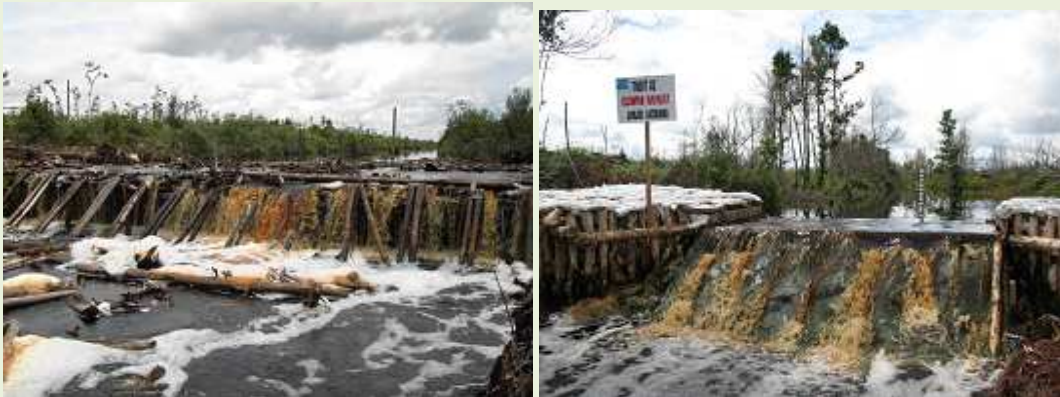
Figure 4: Dams constructed at canal in Block A North, Ex-Mega Rice Project
