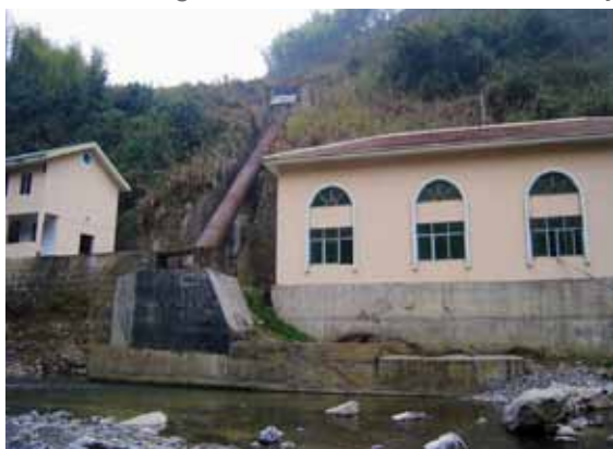
Outside view of Lianghekou hydro plant
