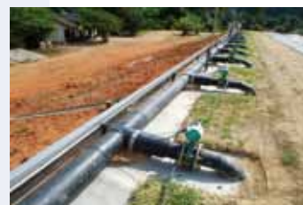
6 Biogas pipeline
